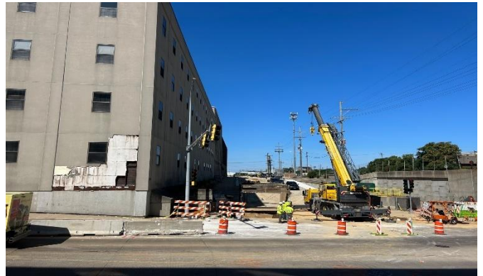
VIEW FROM SITE TO THE WEST
